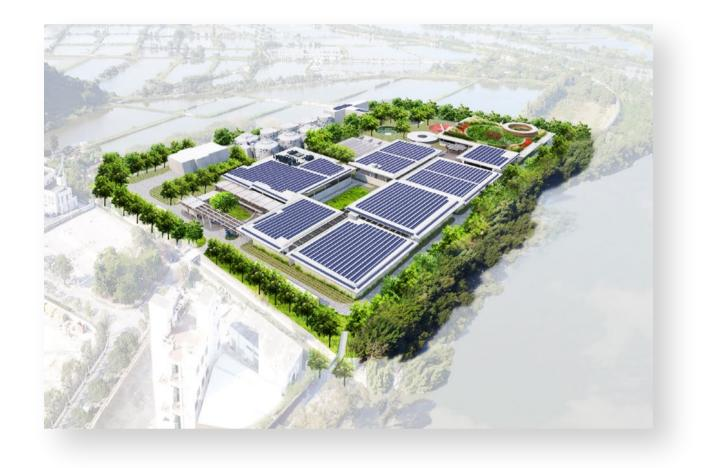
The project is to upgrade the existing Yuen Long Sewage Treatment Works to a tertiary treatment plant within the same footprint. Energy neutrality is achieved in Yuen Long Effluent Polishing Plant through energy saving, utilisation of renewable energy, optimised hydraulic and building design, in pursuit of the Government's goal of achieving carbon neutrality in 2050.
